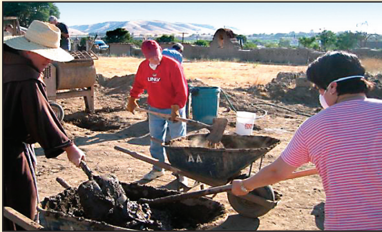
Volunteering to make adobe bricks
